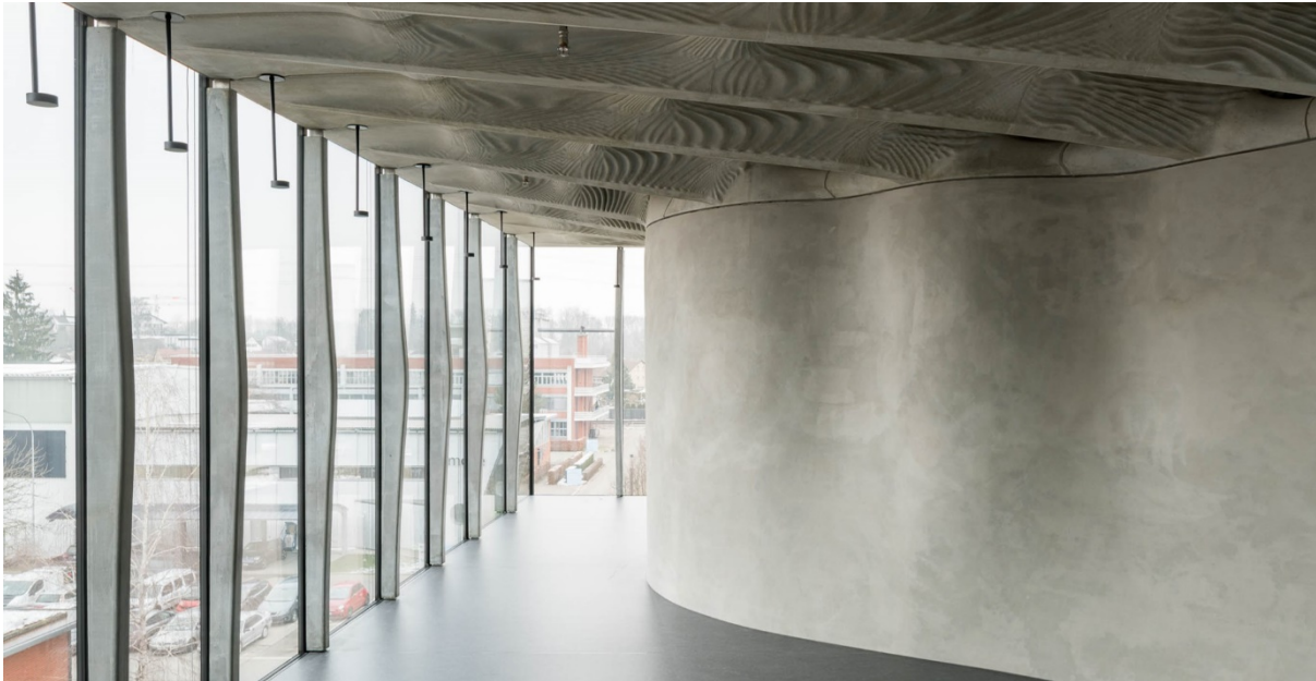
Figure 3. Concrete innovations in the first floor of the DFAB HOUSE: left, mullions produced with the Smart Dynamic Casting technology; right, Mesh Mould double curved wall; up, Smart Slab (photo: Roman Keller).
