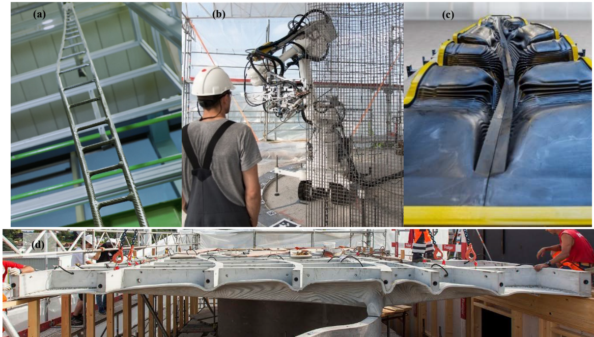
Figure 4. Details of production of concrete structures for the DFAB HOUSE: (a) reinforcement of the mullions installed prior concrete production [92]; (b) onsite robotic fabrication of double curved reinforcing mesh [93]; (c) 3D-printed formwork for a 7.1 m segment of the Smart Slab [94]; (d) installation of the prefabricated Smart Slab [94].
