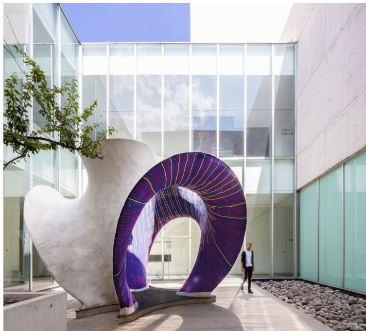
Figure 6. Finished KnitCandela concrete shell showing the soft textile interior and the smooth concrete exterior [99].
