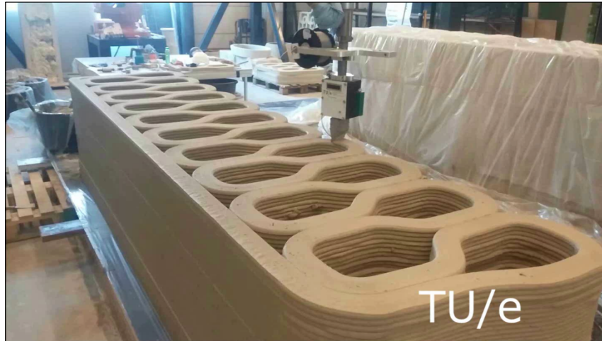
Figure 9: Printing of one of the parts of the bicycle bridge at the 3DCP facility of the TU/e
