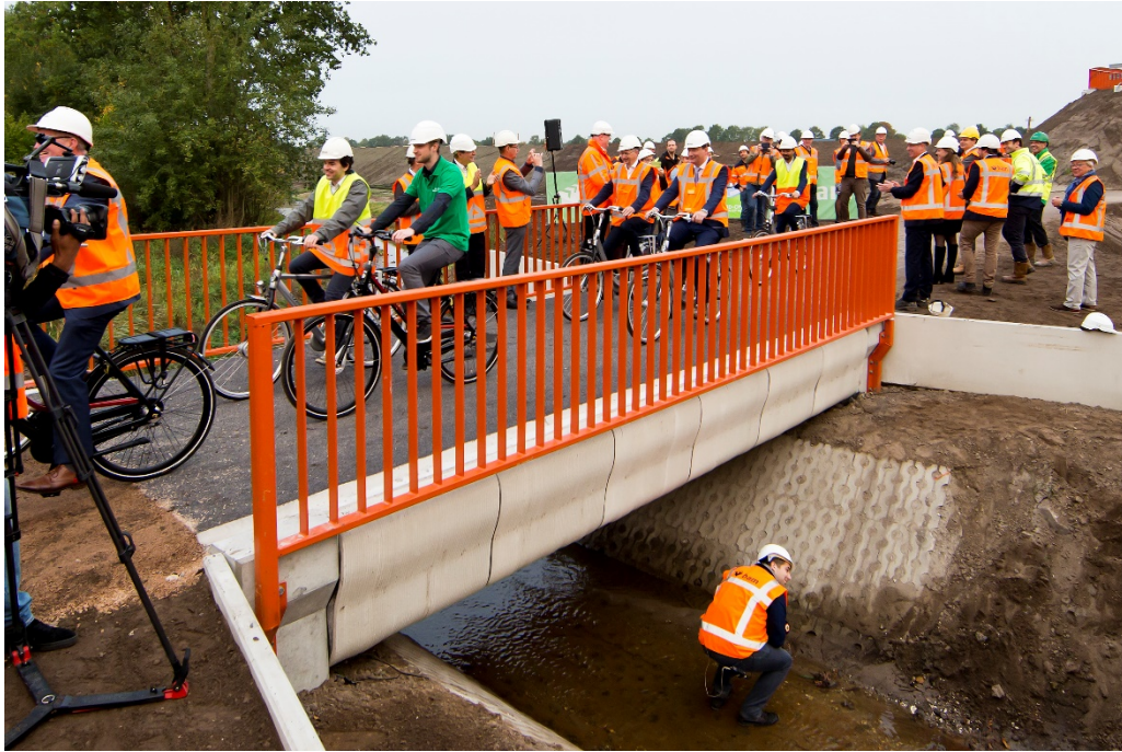
Figure 8: 3DCP bicycle bridge in Gemert, at the opening event in October 2017 (photo: Kuppens Fotografie)
