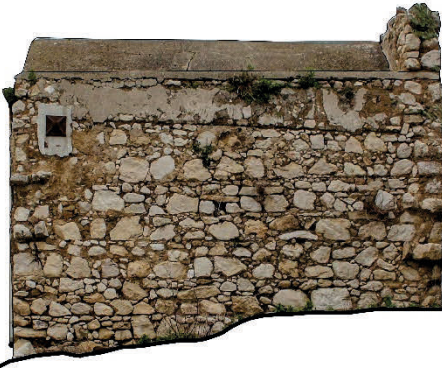
Fig. 4 – East orthophoto of the residential cluster: the masonry with periodic layers (Author, 2025).
