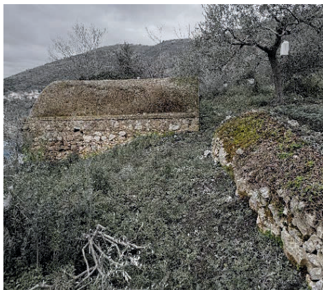
Fig. 2 – Production unit and masonry (Author, 2025).
