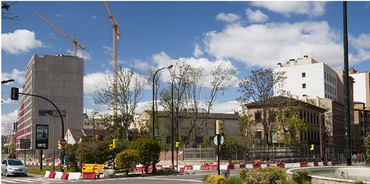
Figure 9. Current view of the Averly foundry among the rubble and the new block of flats under construction. Author: Antonio Duaso Clusa.
