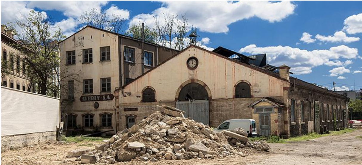
Figure 8. Current view of the Averly foundry among the rubble and the new block of flats under construction. Author: Antonio Duaso Clusa.
