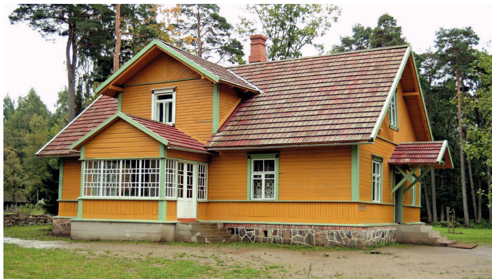
Fig. 7 – A roof of original concrete tiles on the Härjapea farm dwelling relocated to the Estonian Open-Air Museum (Pärdi, 2007).
