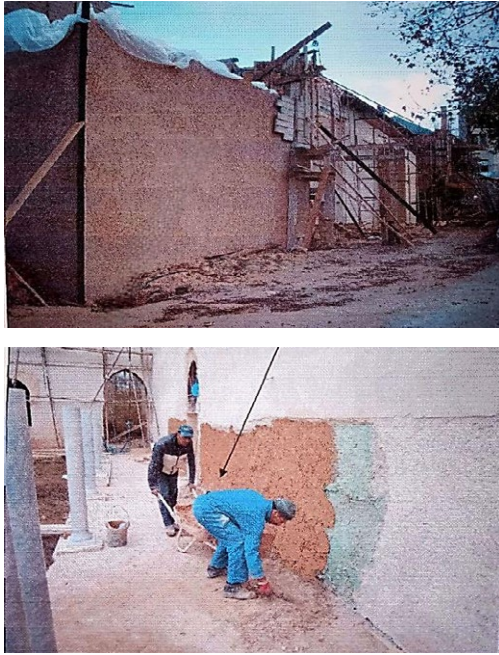
Fig. 8. Wall cladding process. (Source: Technical Design Office A.R.C.A.D.E. 2011).
