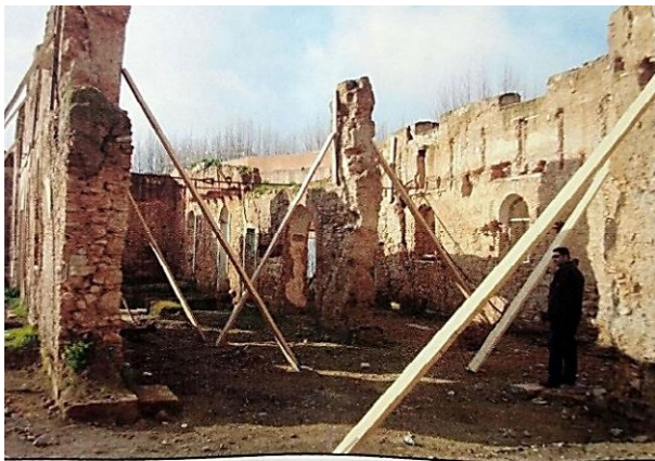
Fig. 6. Wall reinforcement process. (Source: Technical Design Office A.R.C.A.D.E. 2011).
