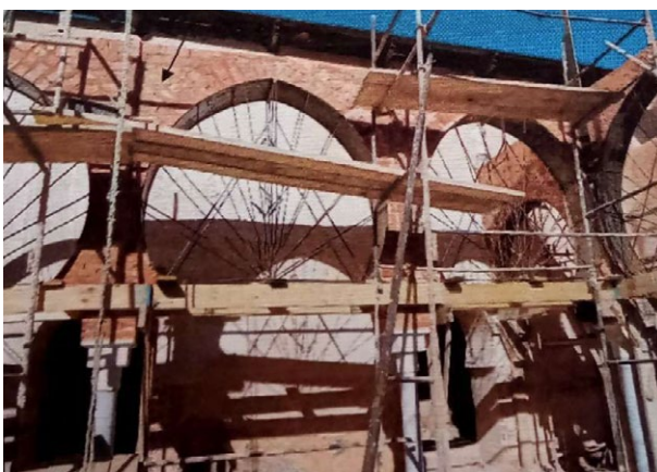
Fig.14. Construction of arches and walls along the arcades. (Source: Technical Design Office A.R.C.A.D.E. 2011).
