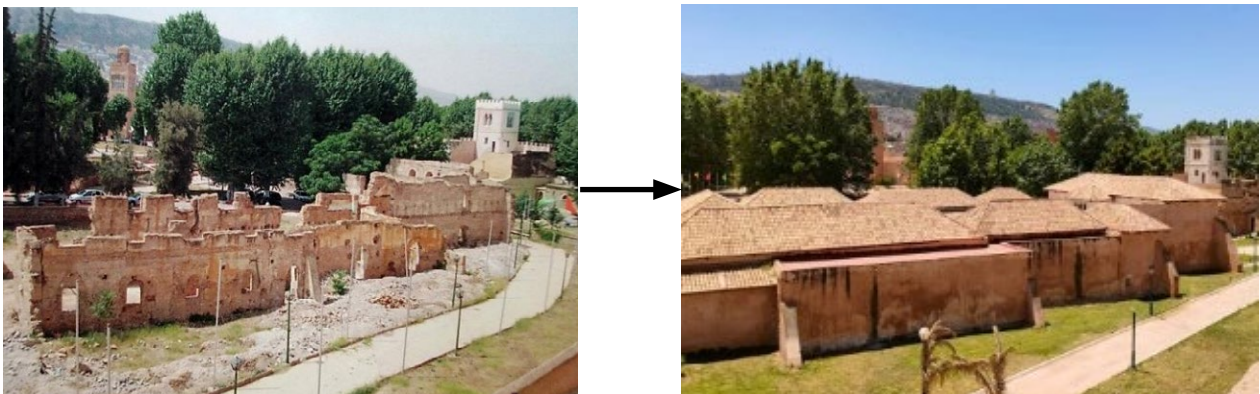
Fig.22. Northern façade before and after reconstruction.
