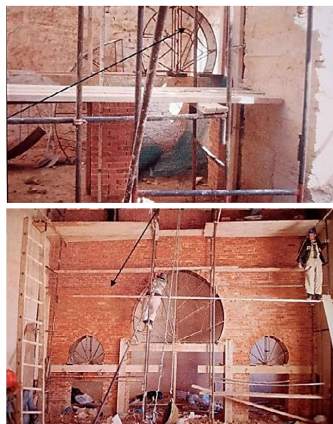
Fig.12. Construction of internal walls and brick arches. (Source: Technical Design Office A.R.C.A.D.E. 2011).
