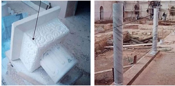
Fig.13. Installation of marble columns supporting capitals along the arcades. (Source: Technical Design Office A.R.C.A.D.E. 2011).
