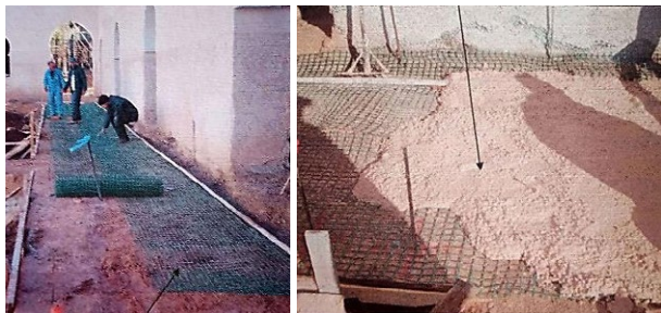
Fig.9. Floor tiling process. (Source: Technical Design Office A.R.C.A.D.E. 2011).
