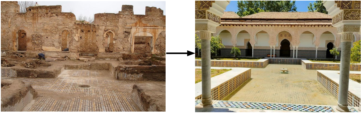
Fig.21. Southern interior façade before and after reconstruction.
