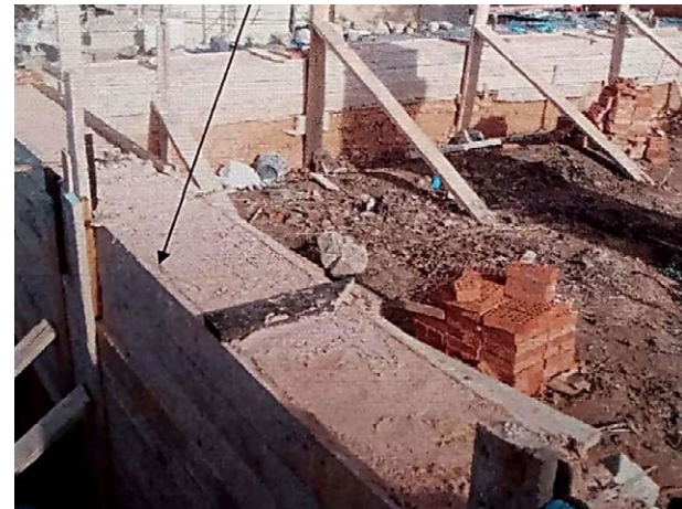
Fig. 7. Placement of formwork for wall construction. (Source: Technical Design Office A.R.C.A.D.E. 2011).
