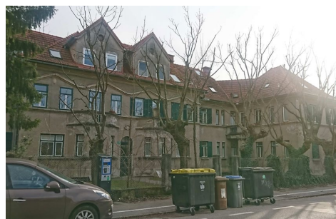
Fig. 2 – View on the north, main façade before renovation (GI ZRMK, 2021).
