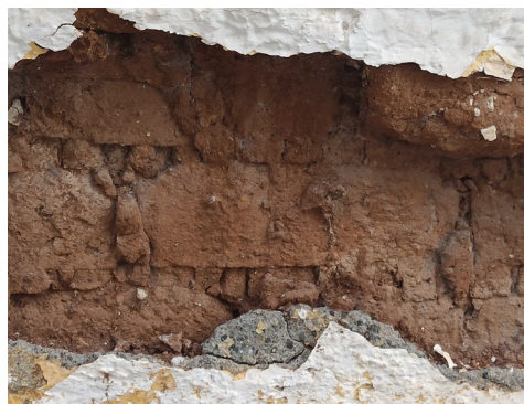
Fig. 7 – Tirana: intervention with cement mortar on qerpiç (Rescic, 2024).
