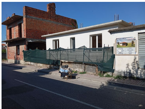
Fig. 11- Kavaje: building completely rebuilt in baked bricks and concrete after the effects of the 2019 earthquake in Fig. 6 (Çapeli, 2024).
