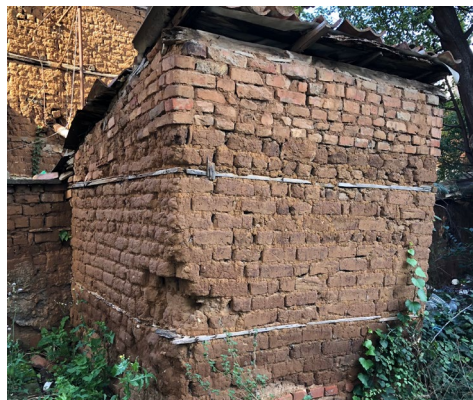
Fig. 5 – Tirana: wall made of qerpiç (sun-dried earthen bricks) and reinforced with horizontal wooden beams, fired bricks are present at the base and below the roof (Luvidi, 2024).
