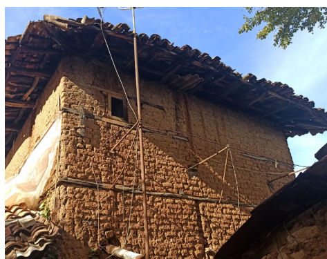
Fig. 6 – Tirana: particular of wooden battens and slightly overhanging roof (Rescic, 2024).
