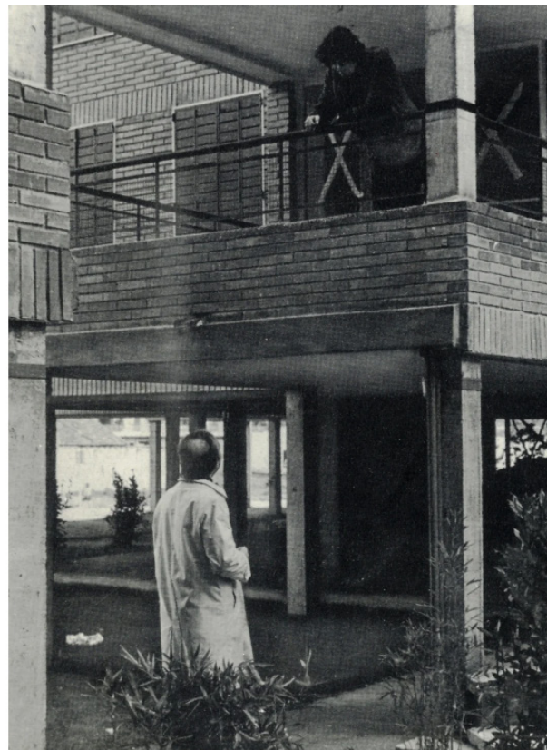
Figure 4 | 1970's photo of Las Fronteras social housing, Torrejón de Ardoz, Madrid. Source: Modulo Hele de Rafael Leoz.
