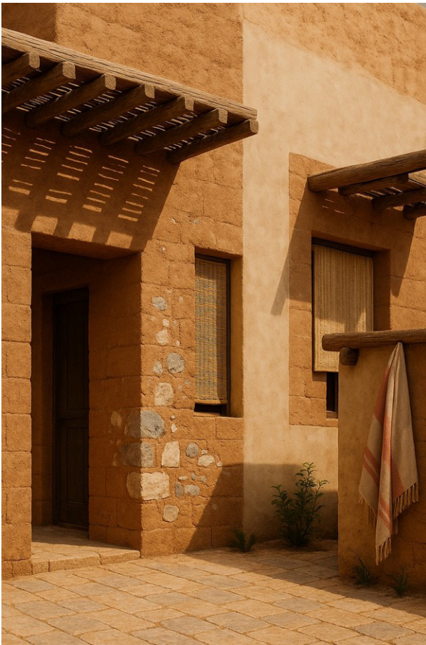
Figure 8 | Material Atmosphere and Texture Study . Close-up rendering of façades and materials, showing compressed earth blocks (CEBs), rubble-based components, lime plaster finishes, and palm wood shading systems. The image illustrates the tactile quality and ecological intelligence of the material strategy.
