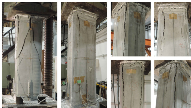
Figure 16. Details of the failure of rectangular columns with b/h = 1.5 .
