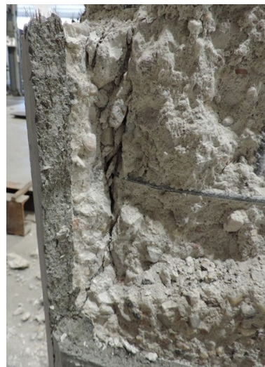
Figure 19. Column tested—good adhesion of the jacket to the substrate.
