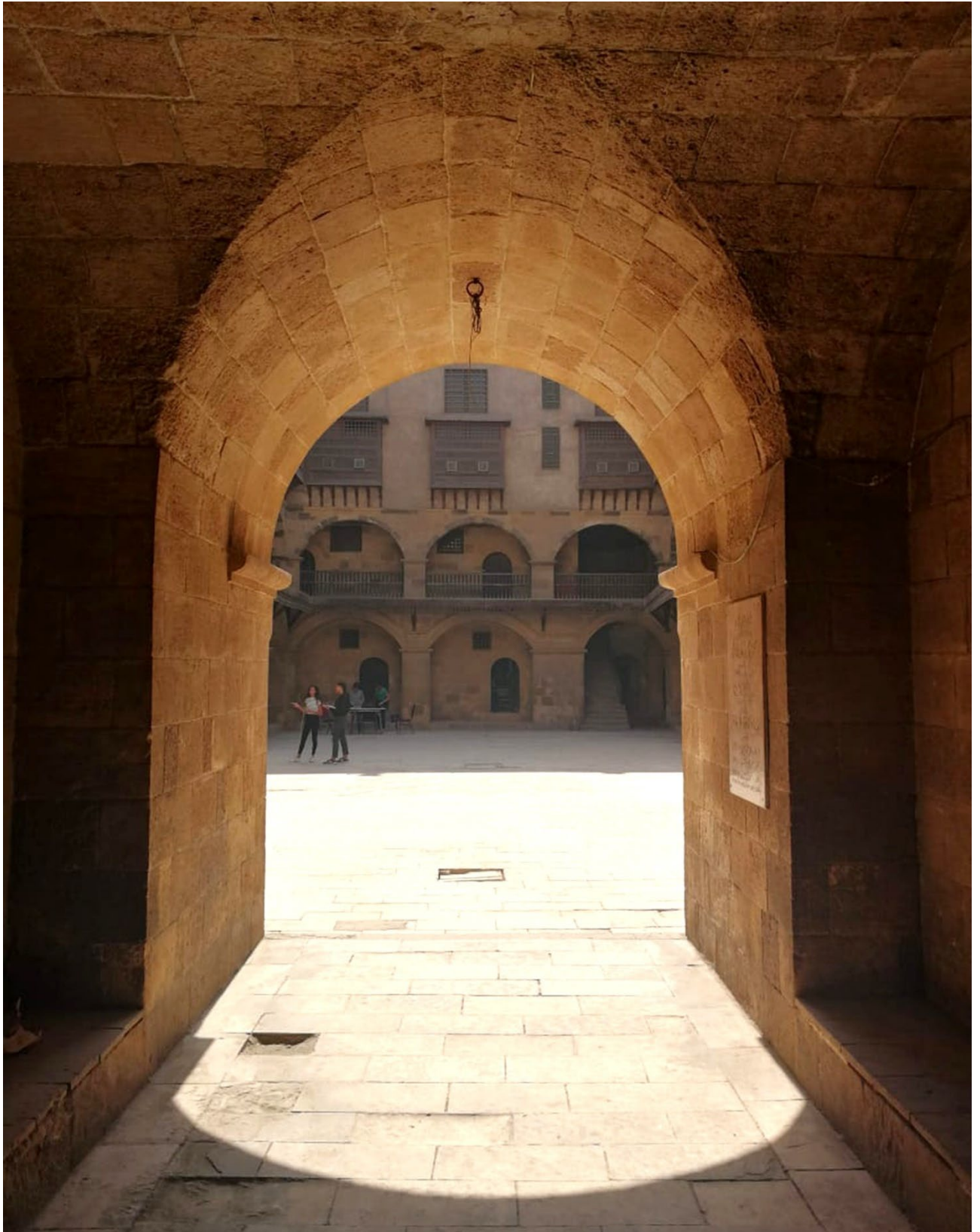
Fig. B2. The vaulted passageway of Wekalet Bazaraa leading to the central courtyard, showing how the narrowing and widening of space guides airflow and creates a micro-cooling effect through compression and release. Photograph by Lamiaa Ghaz, 2019, used with permission.
