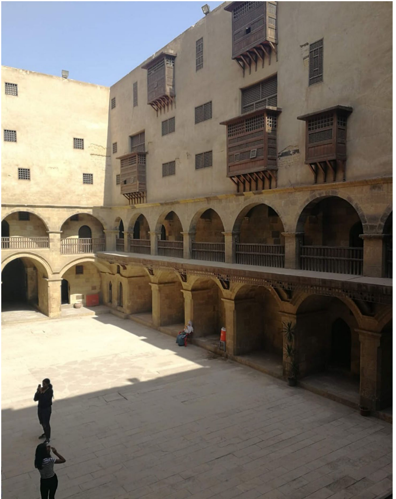
Fig. 12. Courtyard of Wekalet Bazaraa showing arcaded thresholds on the ground floor and shaded corridors on the first floor. Source: Photograph by Lamiaa Ghaz, used with permission.
