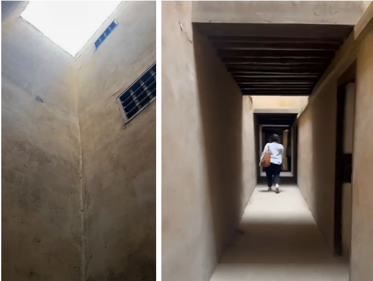
Fig. 19. Light wells and their effects along the upper residential corridor. Left: view looking up through the vertical shaft admitting daylight. Right: corridor illuminated by the light wells, with a solid eastern wall ensuring privacy and insulation from the neighbouring building without sacrificing natural light. Source: Author's own photos.
