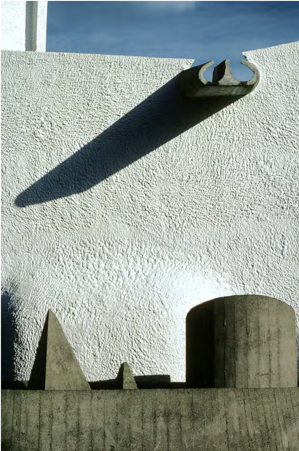
FIG.54 Le Corbusier, Millowners' Rochamp, view of rear side with water spout and basin with pyramidal elements to collect and splash water off the roof. The secret and enigmatic life of forms covering layers of hermetic meaning. Photo WJRC, 1986.
