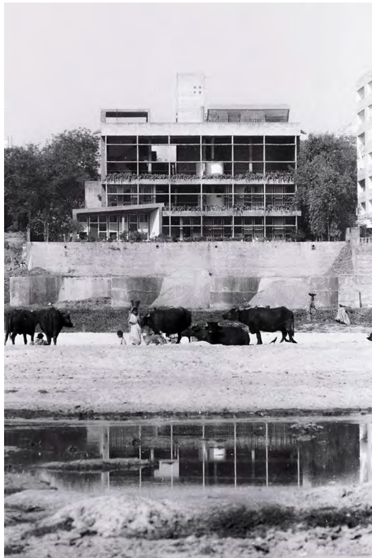
FIG.26 Le Corbusier, Millowner's Association Building, Ahmedabad, India, 1951-54, view across the River Sabarmati to the east façade with its grille of brise-soleil. This view was taken over forty years ago when the river bed was still used for drying dyed textiles and there were oxen and people wandering along its gravel banks. Today the river has become a dead lake, and a concrete walk way cuts off the building from the water. Photo WJRC, 1984.
