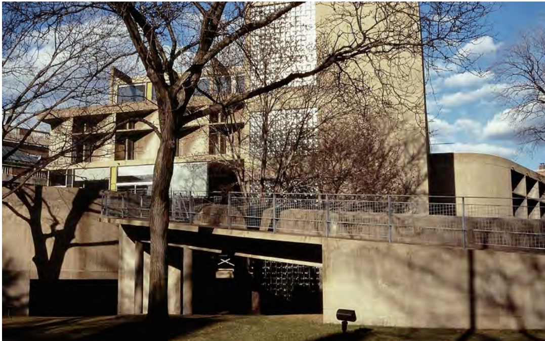
FIG. 11 Le Corbusier, Carpenter Center for the Visual Arts, Harvard University, Cambridge, Ma., USA, 1960-62. Front, west side, facing onto Quincy Street. The dynamics of architectural form and space. Photo WJRC 2010.
