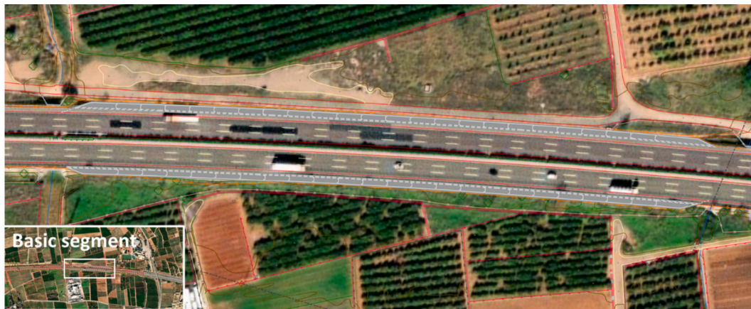
Fig. 11. ERL along a basic freeway segment, located between two drainage systems.
