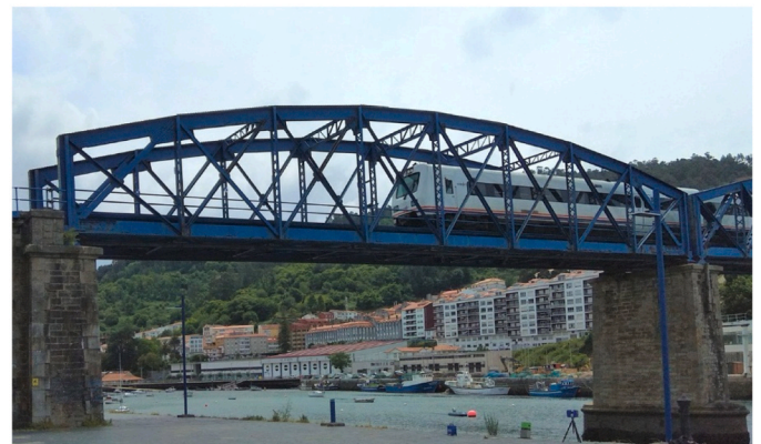
Fig. 2. The steel truss bridge.
