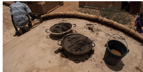
Fig. 7 – Earth tubes installation test (ph. R. Pennacchio).
