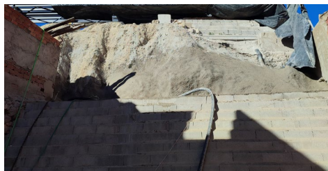
Fig. 8 – Terrain stabilization solutions.
