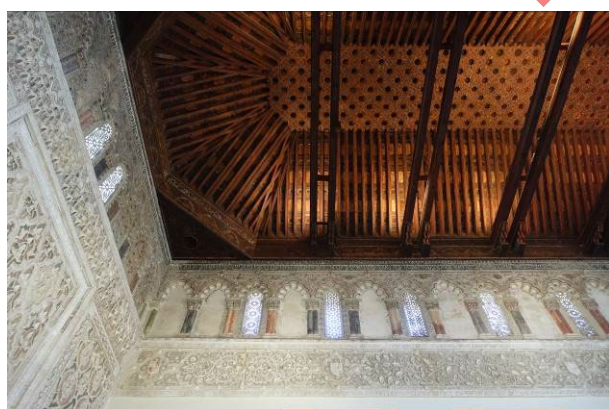
Figure 7: Detail of the semi-hexagonal finishing of the coffered ceiling.
