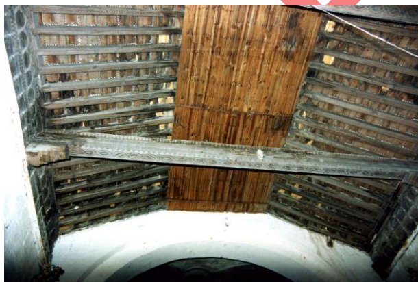
Figure 19: coffered ceiling of the parish church of Almenara de Tormes (Salamanca).
