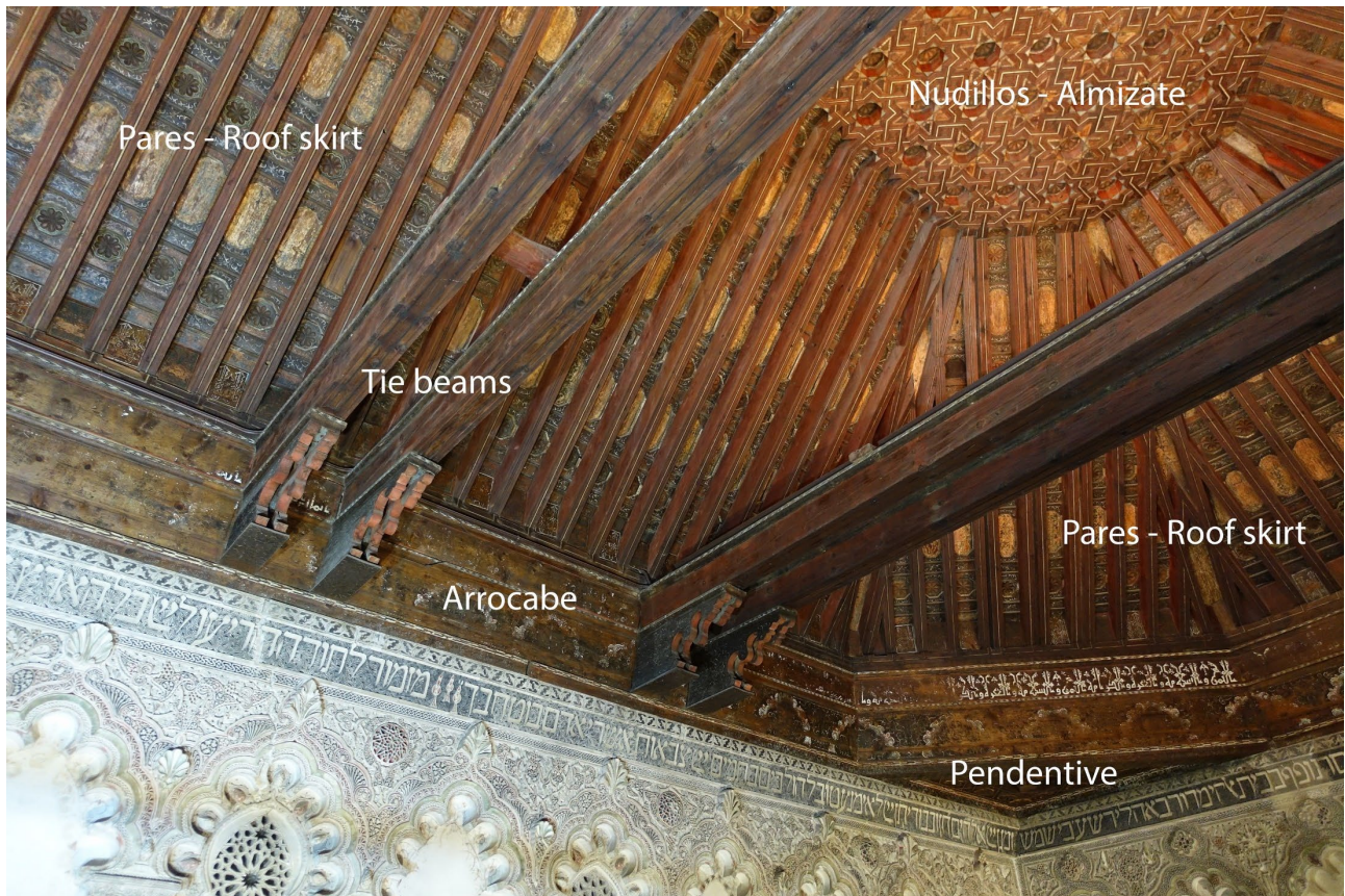
Figure 17: Coffered ceiling with its main constructive elements.
