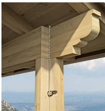
Fig.35 Simplex, section illustration [Rothoblaas, 2024]
