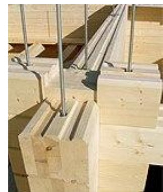
Fig.37 Construction photograph [Casalt, 2011]
