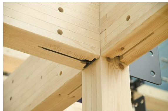
Fig.60 Joint photograph [Xiaofu, 2019]
