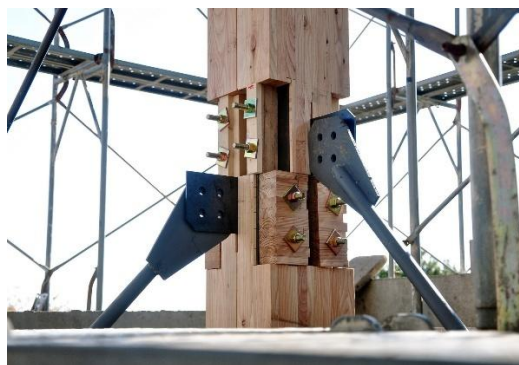
Fig.97 Detail photograph during construction [UC Berkeley CED graduate team, 2014]
