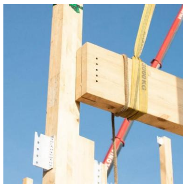
Fig.62 Construction photograph [Azalea UPV, 2022]
