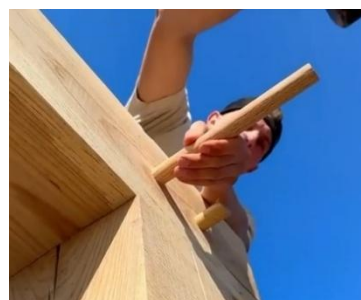
Fig.14 Construction photograph [Worzalla Brothers, 2024]
