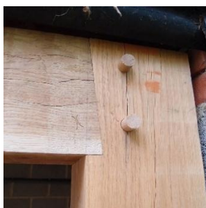
Fig.13 Joint photograph [Aires, 2025]
