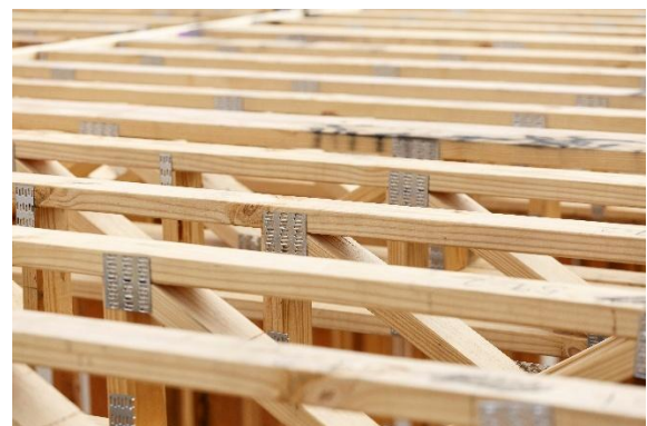
Fig.56 Joint photograph [Westbrook, 2013]
