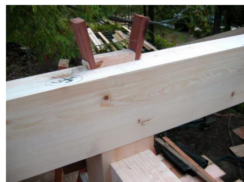
Fig.26 Construction photograph [TRC Timberworks, 2025]
