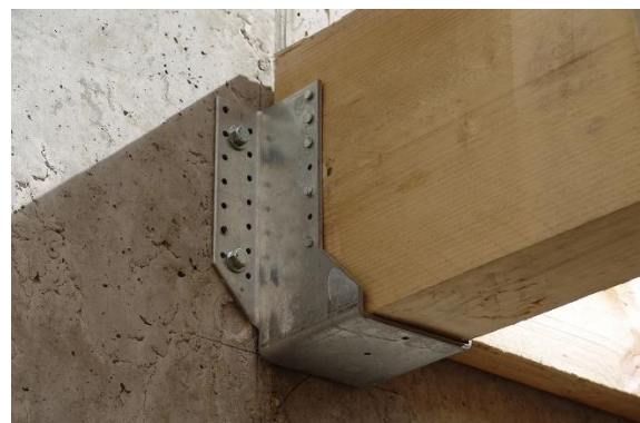
Fig.79 Timber to concrete joint [Sobrico, 2025]
