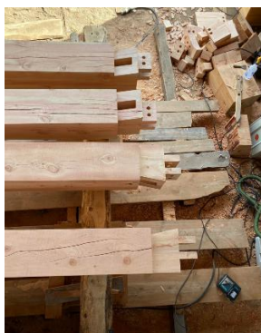
Fig.24 Construction photograph [u/angry_timberframer, 2023]
