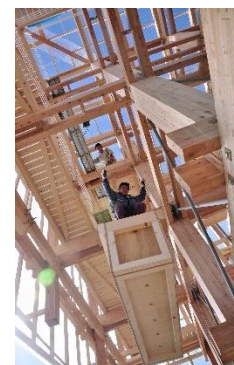
Fig.100 Photography during construction [UC Berkeley CED graduate team, 2014]
