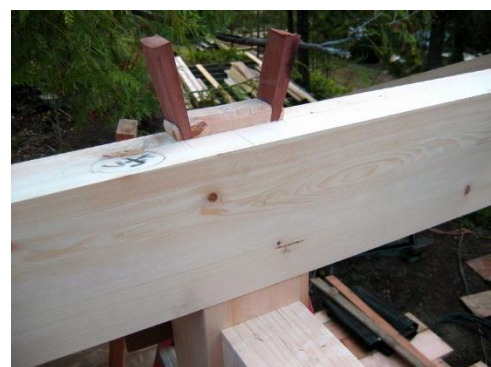
Fig.26 Construction photograph [TRC Timberworks, 2025]
