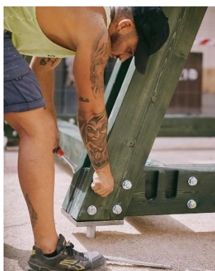
Fig.44 Mediterráneo Pavilion construction photoraph [Bouzas, 2023]
