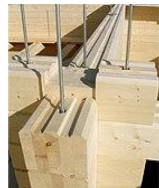
Fig.37 Construction photograph [Casalt, 2011]
