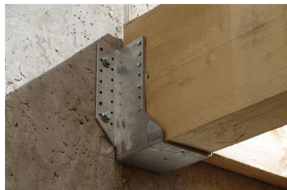
Fig.79 BSI timber to concrete joint [Rothoblaas, 2024]
