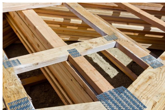
Fig.54 Construction photograph [Stock, 2014]
