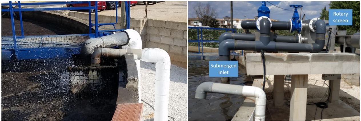
Figure 2. Views of the bioreactor inlet pipe: (a) open-air inlet discharging directly onto the bioreactor screen during the first measuring campaign: (b) submerged inlet to avoid splashing and the release of dissolved gases during the second measuring campaign.
