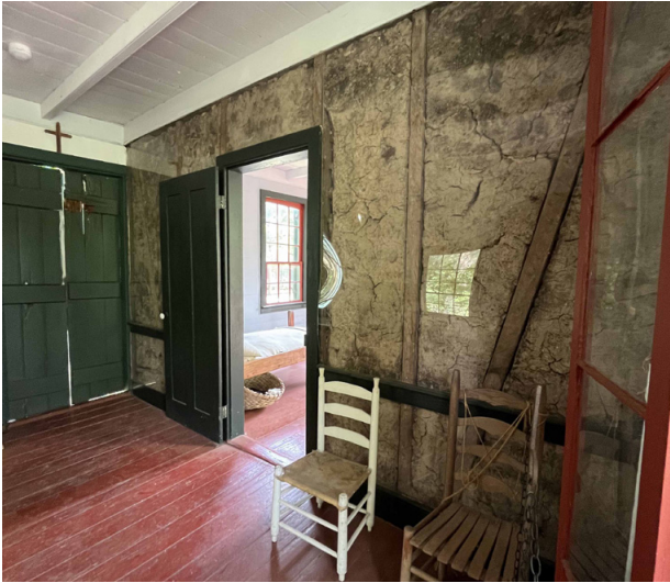
Figure 7 | Interior walls made by bousillage of SM in the village of Vermilionne (credit: author, 2023).
