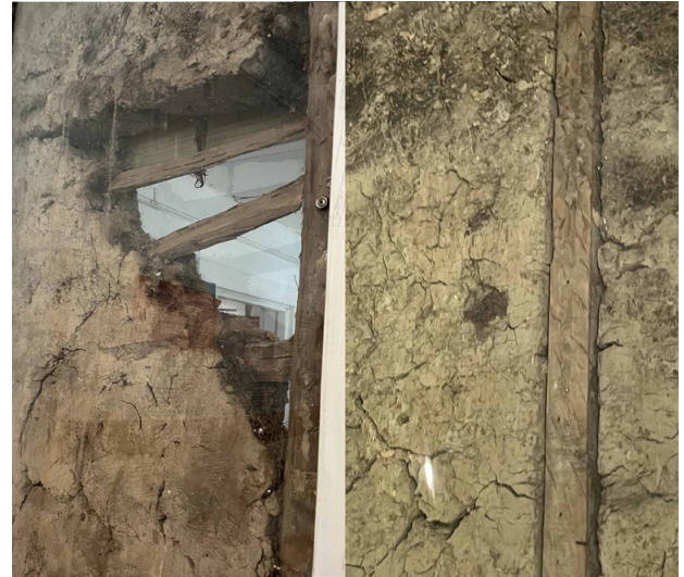
Figure 8 | X-ray of the wooden substructure with the insulating fill of mud and SM in Vermilionne (credit: author, 2023).
