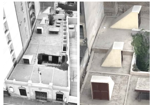
Fig. 1 – Aerial photography and Teatinas on the roof (Díaz, 2024).
