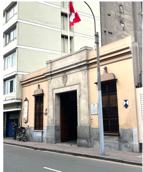
Fig. 2 – Facade of the study building (Díaz, 2024).
