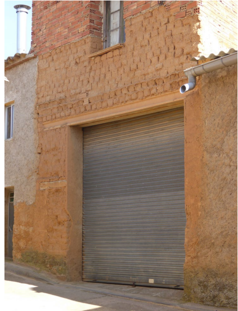
Fig. 4 – Adobe wall where the entrance has been enlarged (Vegas & Mileto, 2016).
