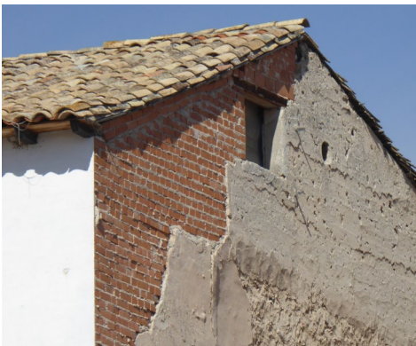
Fig. 3 – Rammed earth wall intervened with industrial brick (Vegas & Mileto, 2016).
