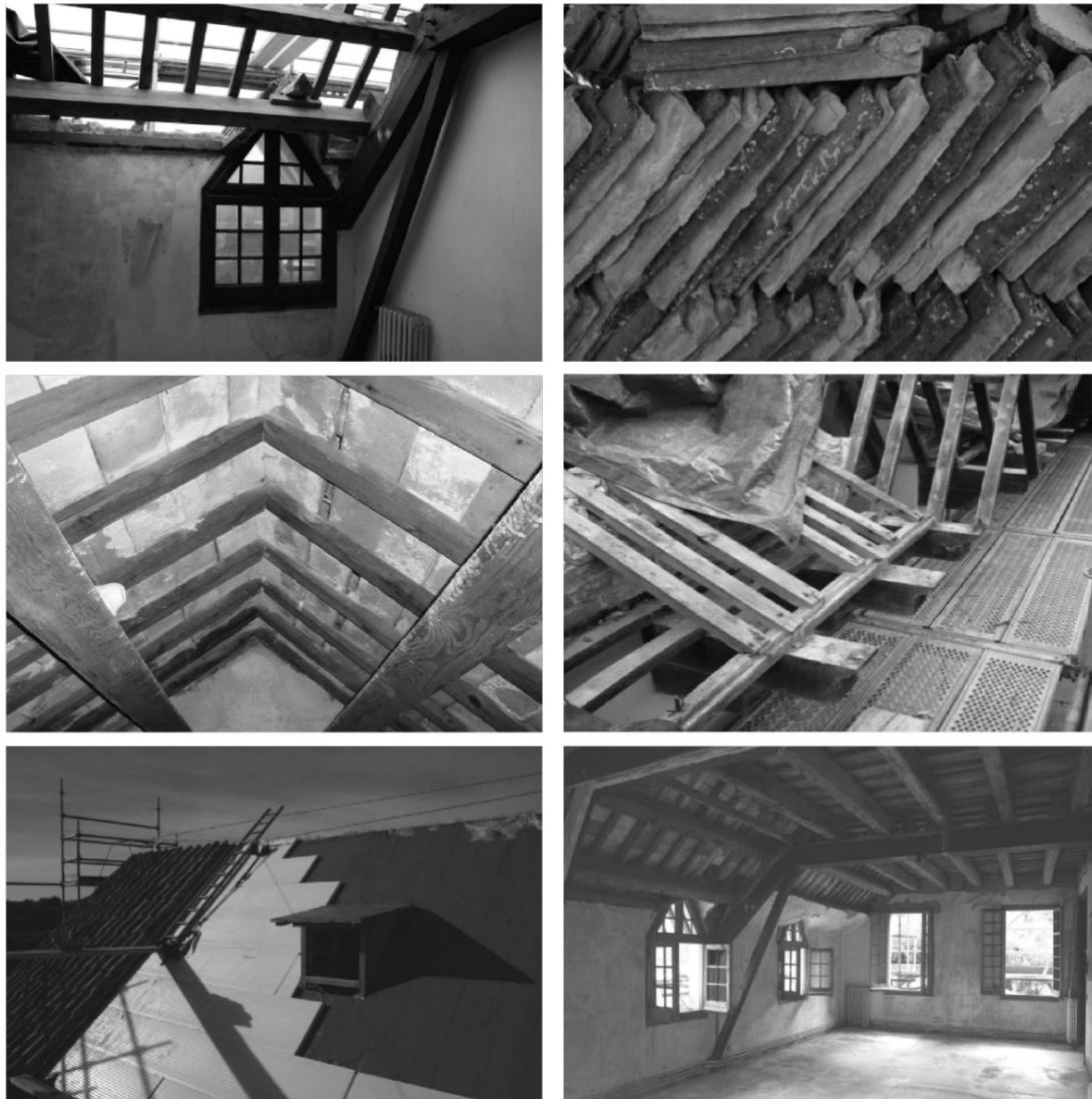
Figure 6 | Taken by the author. Process of retrofitting the roof at Casa Pilar Moragas.
