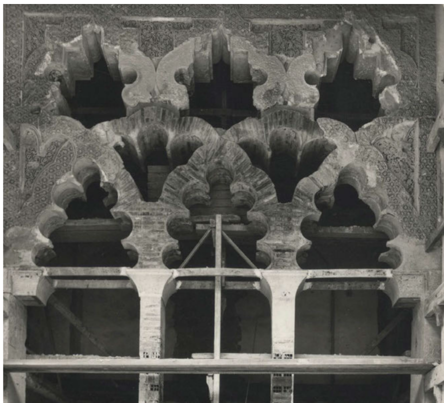
Figure 4. Patio de Santa Isabel. South Side Door. Source: Iñíguez Almech, F. 1968. AGA (General Administration Archive), Signature 26/00214.
