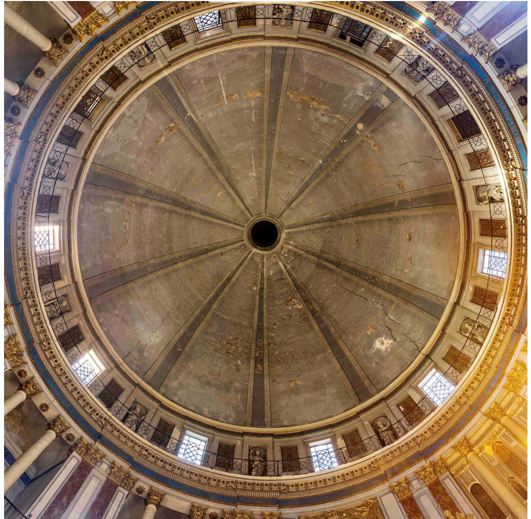
Figure 3. View of the dome and the cracks in four different sectors.
