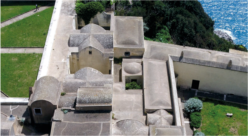
Fig. 4 – Extrados vaults of Chartreuse of San Giacomo in Capri next to the Quart of Prior (Facchini, 2018).
