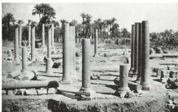
Figure 8: Ruins of the Basilica Church (1949). Photo after Wace et al., 1959, pl. 20, Fig. 2.
