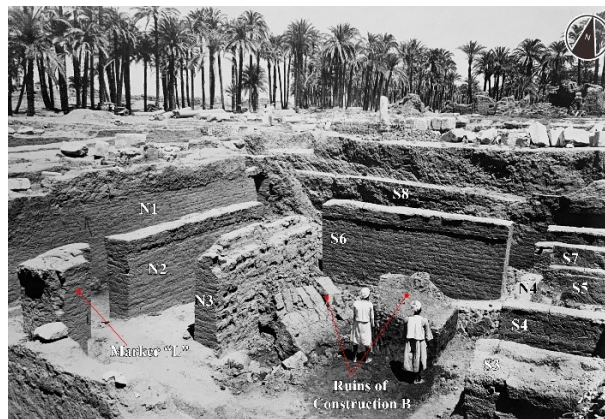
Figure 19: Post-demolition view of the area underneath the atrium; S2 and construction B are demolished/in ruins (BM REF: 24). Photo © The Trustees of the British Museum. Available under a Creative Commons CC-BY-NC-SA 4.0 Licence.
