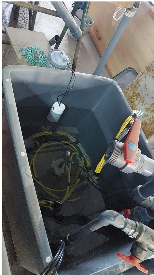
Fig. 9. Battery duration experiment during EU H2020 SMARTLAGOON project assembly.
