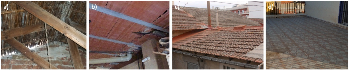
Fig. 6. a) Timber roof truss with "cañizo", b) Slab made of reinforced concrete frames with ceramic vaults, c) Sloping roof with ceramic shingles, d) Flat roof with ceramic tiles (Image credits: Valencia Institute of Building, IVE).
