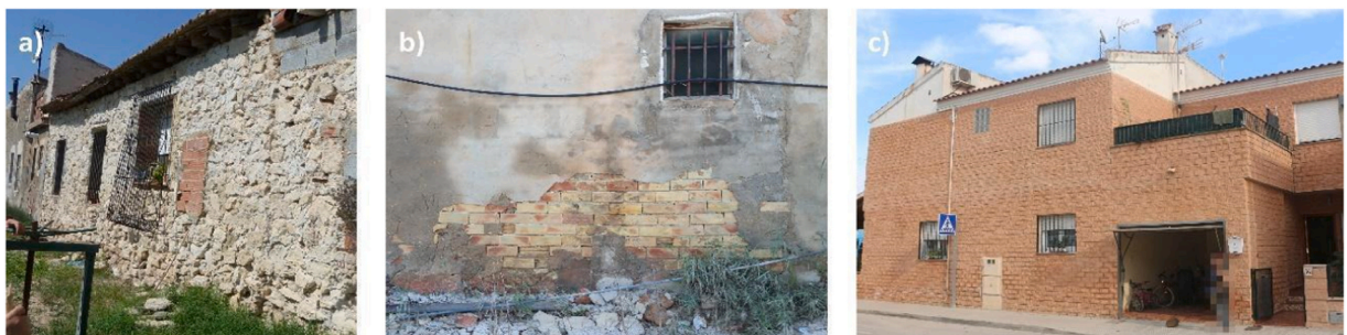
Fig. 5. a) Rubble masonry fabric, b) Brick masonry fabric, c) Concrete block masonry fabric (Image credits: Valencia Institute of Building, IVE).
