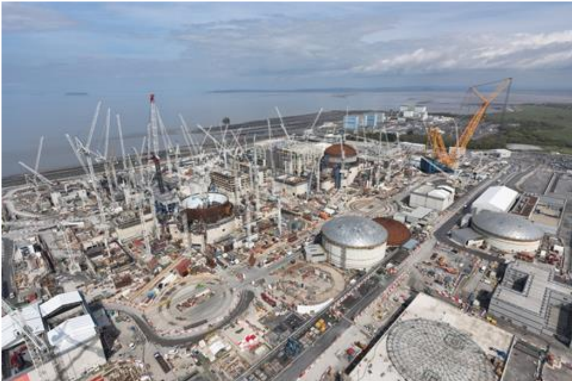
Figure 9. Hinkley Point C in construction
