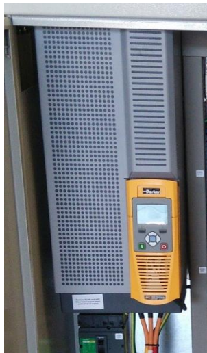
Figure 3.13 – Parker AC30V inverter in the altitude simulator
