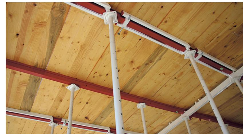
DETALLE DEL SISTEMA ALUMECANO
