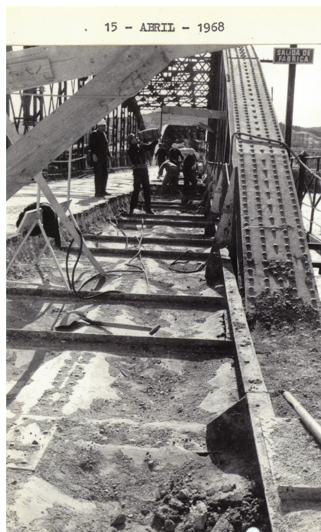
Figure 3. The repair of the year 1968
