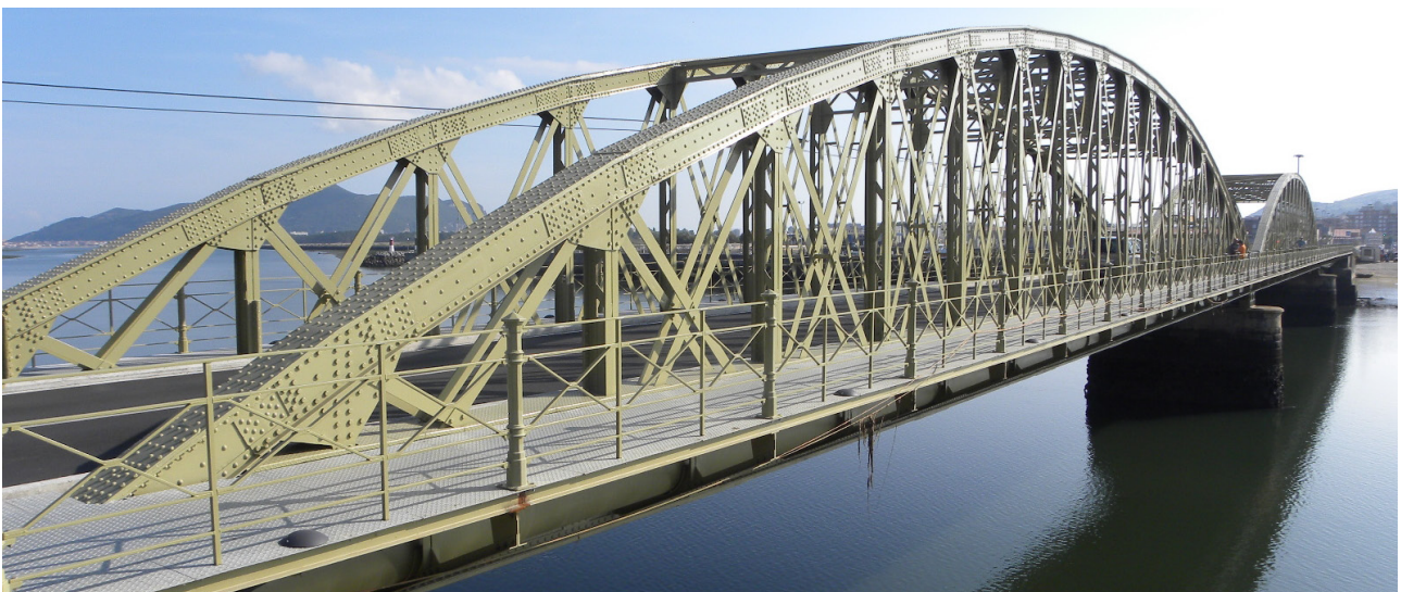
Figure 10. Current status of the refurbished stretches
