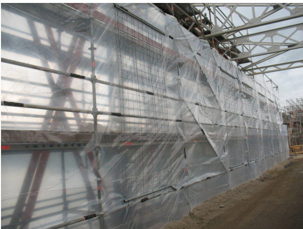
Figure 6. View of the encapsulated scaffold
