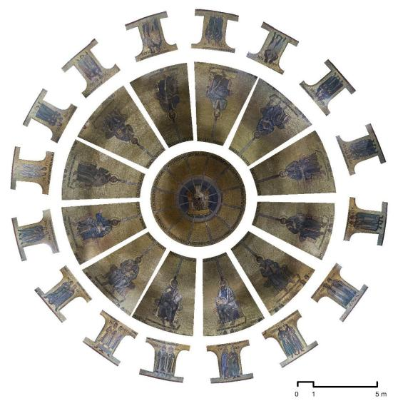
Figure 12: The Dome of Pentecost, subdivided into smaller orthophoto details.
