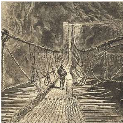
Figure 5 Fibrous suspension bridge
