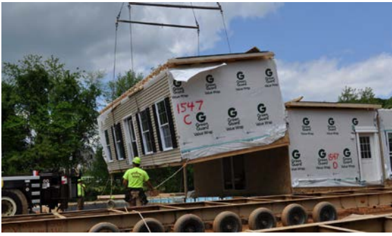
Fig. 9. Unstable module during assembly [13].
