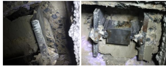
Fig. 14. Bottom view, slide of steel profile, Cv2.
