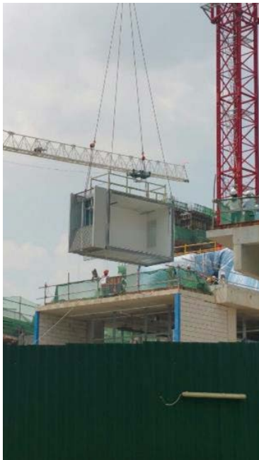
Fig. 11. Locating the module.
