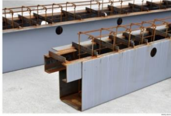
Fig. 4. U Shaped Concrete-Steel Hybrid Beam
