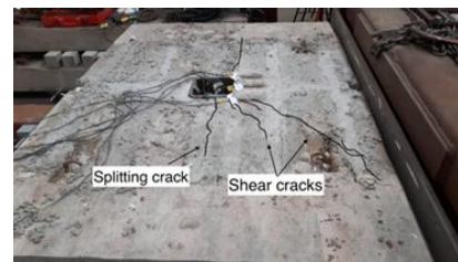
Fig. 10. Cracking pattern of slab of SP5
