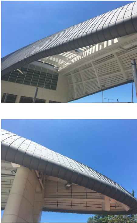
Fig. 3. Triangular shape structure of Kennedy Town Swimming Pool Phase II.
