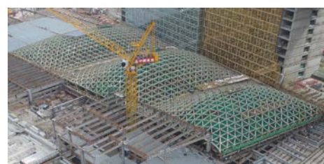
(a) Overall view
