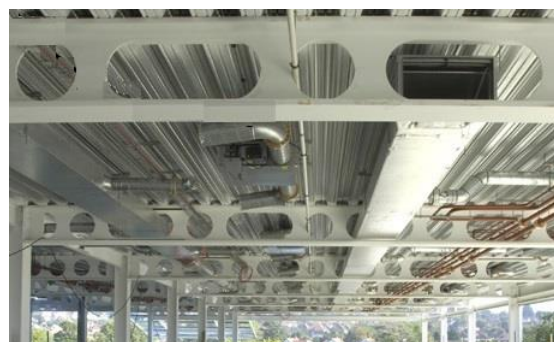
Fig. 1. Cellular beams with regular openings.
