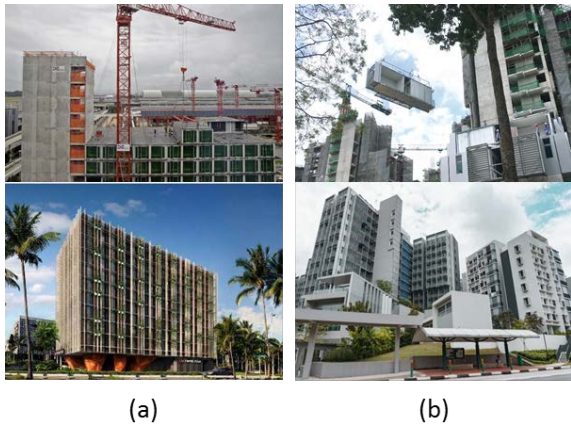
Fig. 1. Pioneer PPVC projects in Singapore (a) Crowne Plaza Hotel Ext @ Changi Airport, and (b) NTU North Hill Residence Hall.
