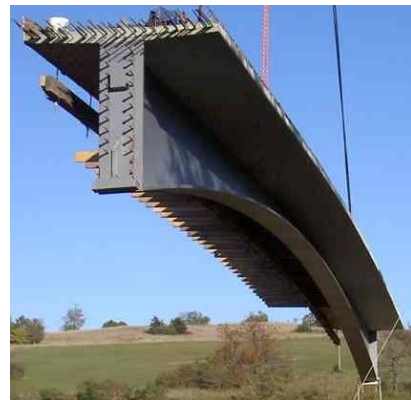
Fig. 1. Prefabricated composite bridge girder with horizontally lying studs [2],[3]
