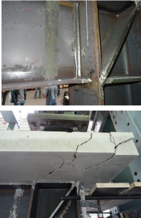
Fig. 4. Observed damage at failure.
