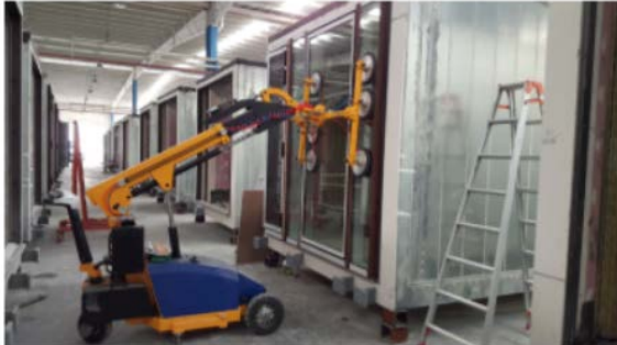
Fig. 12. Interior fit-out in factory [15].
