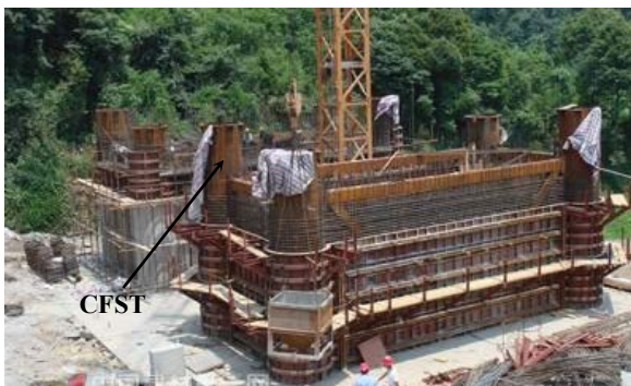
(a) During construction
