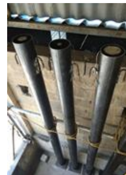
Fig. 3. Concreting of specimens.
