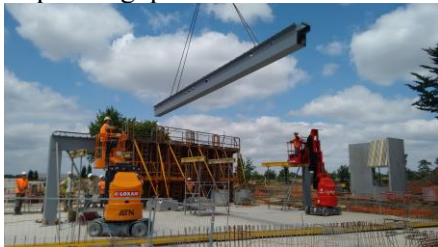
Fig. 27. Erection of the steel portal frame
