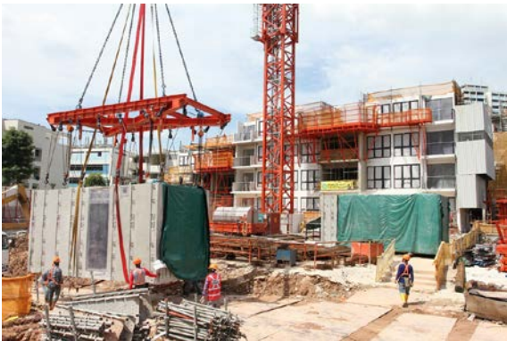
Fig. 10. Lifting of concrete PPVC module [14].
