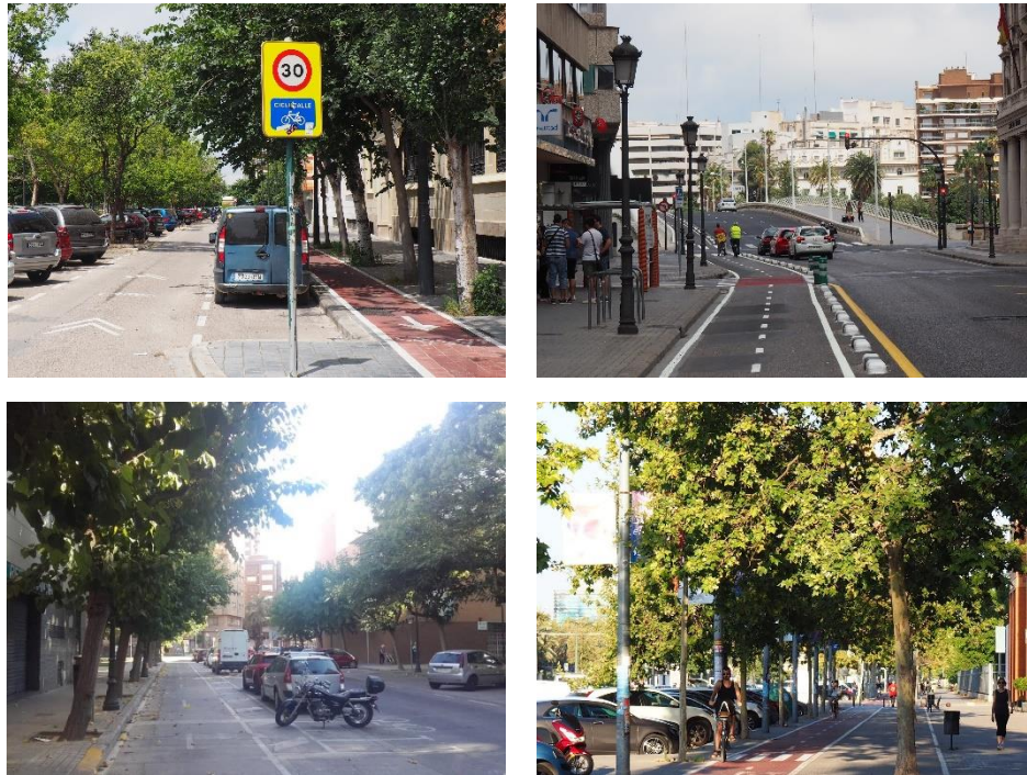
Figure 26: Typical cycling infrastructure in Valencia Top left - Ciclocalle (cycling street) with contraflow one-way cycle path and 30 km/h speed limit Top right - Two-way separate cycle path on a one-way street with two lanes (car and bus lane) Bottom left - Two-way bike path separated by a parking lane from the car lane Bottom right - Two-way cycle path and wide sidewalk next to a four-lane avenue
