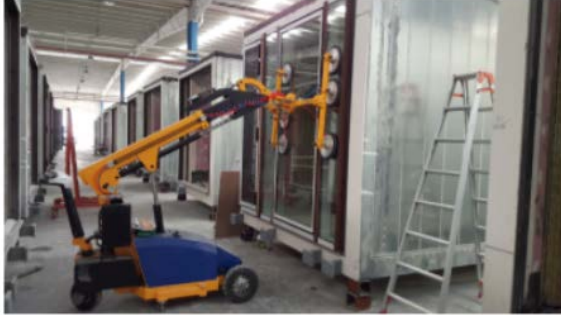
Fig. 12. Interior fit-out in factory [15].
