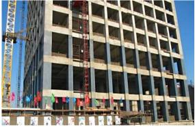
*Fig. 1.* A buildings using STCRC columns in the bottom three stories [1]
