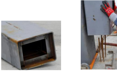
Fig. 26. Column shoe connection
