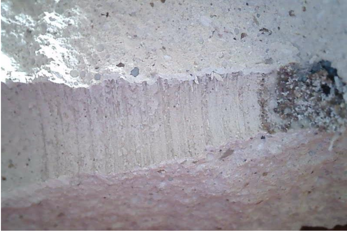
Figure 34: Mould of the top of the tower
