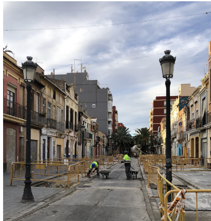
[Fig. 54] On going rehabilitation work, Carrer de la Barraca, 2018, Author
