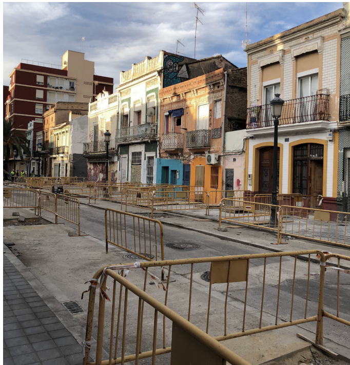
[Fig. 53] On going rehabilitation work, Carrer de la Barraca, 2018, Author
