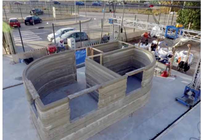
Figura. 1 Modelo teórico y real de casa impresa 3D . BEMORE3D. 2017 / Figure 1. Theoretical and real model of printed house 3D. BEMORE3D. 2017.
