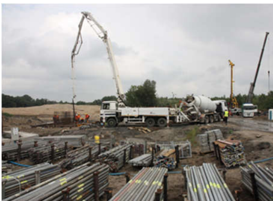
12.07.2018 MG04-01 – P4L concreting of strip footing
