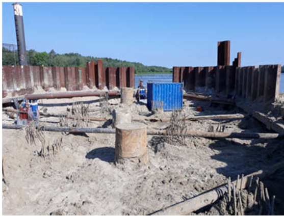
06.07.2018 MG04-02 - P10L - assembly of struts
