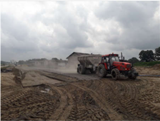
12.07.2018 Ł2 0+120-0+240 – execution of layer of hydraulically bound mixture
