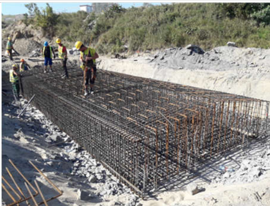
05.07.2018 MG04-01 - P3P – reinforcement of strip footing
