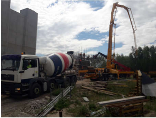
03.07.2018 MG04-01 - P8P- concreting of pier stage I
