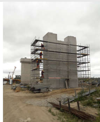
02.07.2018 MG04-01 - P8L – disassembly of scaffolding
