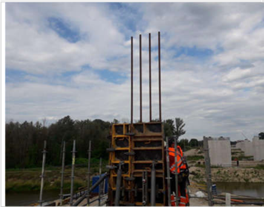
03.07.2018 MG04-02 - 12L assembly of dywidag in props
