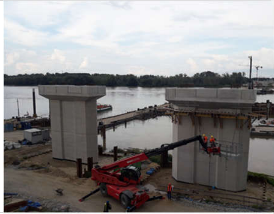
24.07.2018 MG04-01 - P9P removal of formworks of pier
