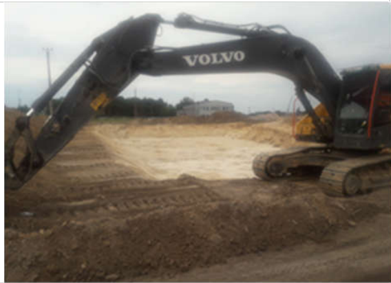
10.07.2018 tank 19A- excavation
