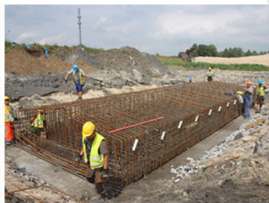
12.07.2018 MG04-01 – P3L reinforcement of strip footing
