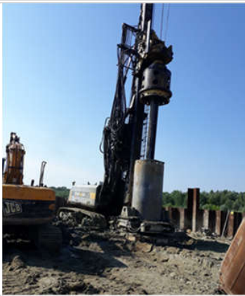
06.07.2018 MG04-02 - P10P – drill hole of pile n0.23
