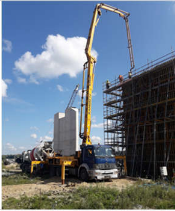
26.07.2018 MG04-01 - P8P – concreting of pier stage II
