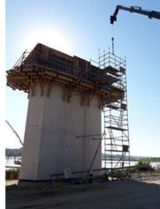
04.07.2018 MG04-01 - P9P – formwork of head
