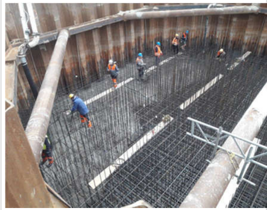
02.07.2018 MG04-02 - 12P – concreting of strip footing stage
