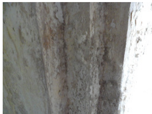
Interior entrada cripta
