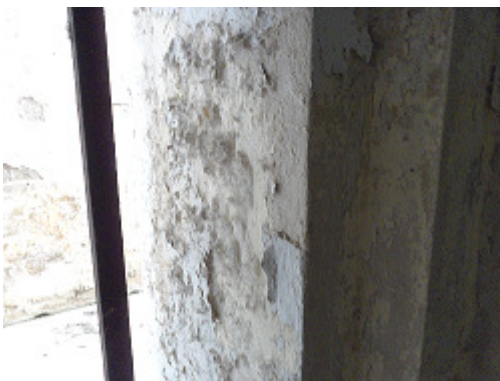
Interior entrada cripta
