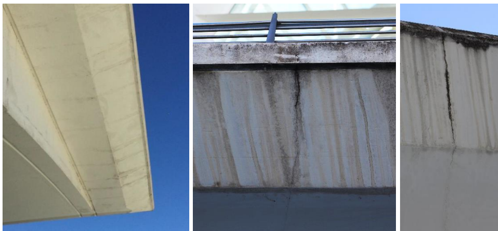
Fig.14. Cracked cornices
