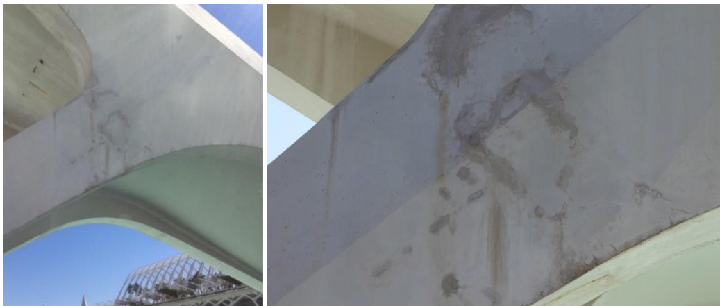
Fig. 20. Patching of concrete surfaces
