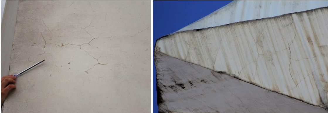
Fig.17. Map cracking
