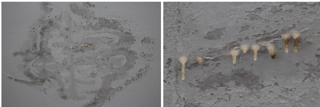
Fig. 10. Calcium carbonate deposits in the form of “stalactites”
