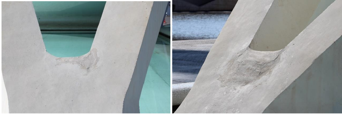
Fig. 21. Repairs with mortar on inter-column joint
