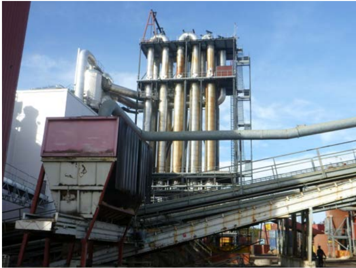
Fig. 1 The five 20m high heat tube shells.
