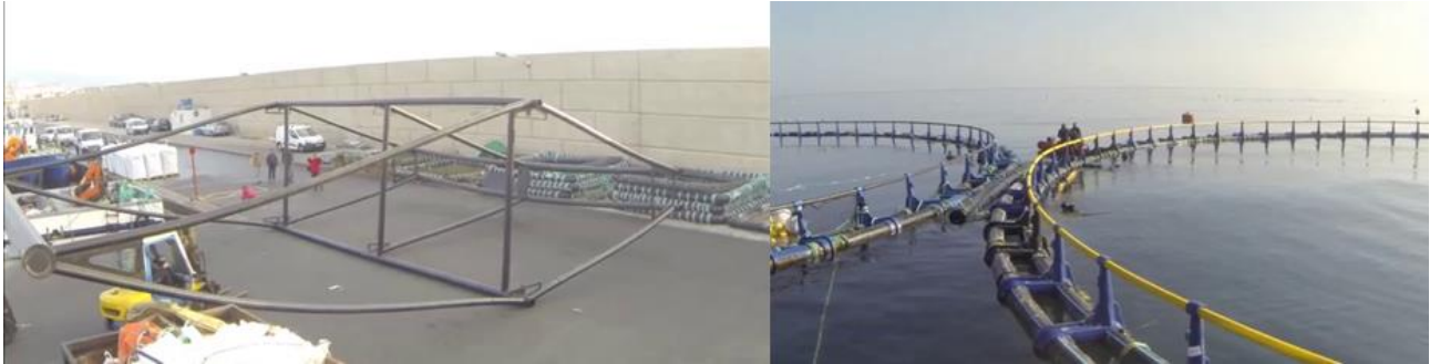
Figure 6. Left, the S3 floating structure on the quay of the port ready to be transported to the cages. Right, surface view of its position between two cages during transfers.
