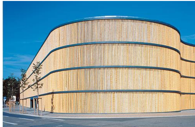
Parking Garage of the Leipzig Zoo. HPP Architects
