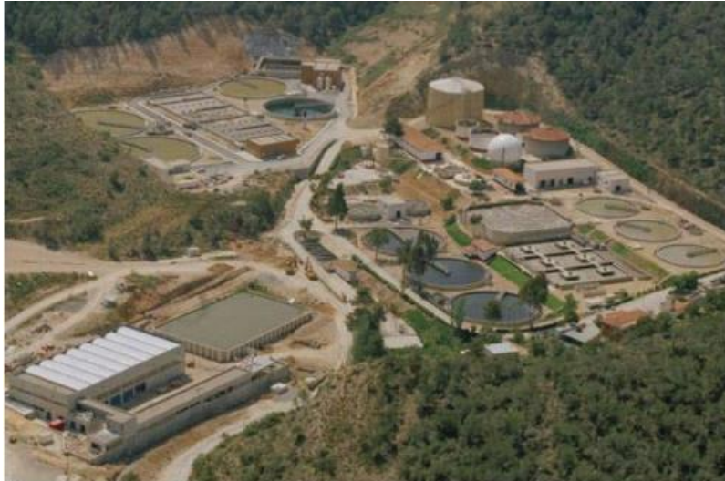
Figure 13. Benidorm Sewage Treatment Plant. [28]
