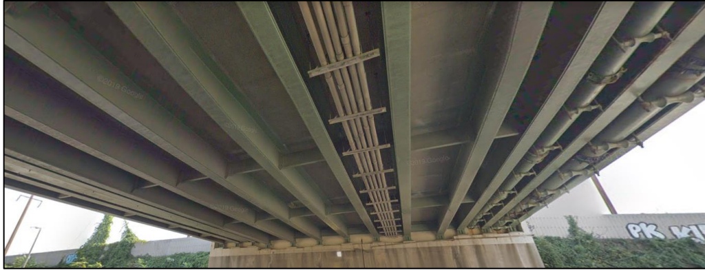
Figure 64. Superstructure of bridge.
