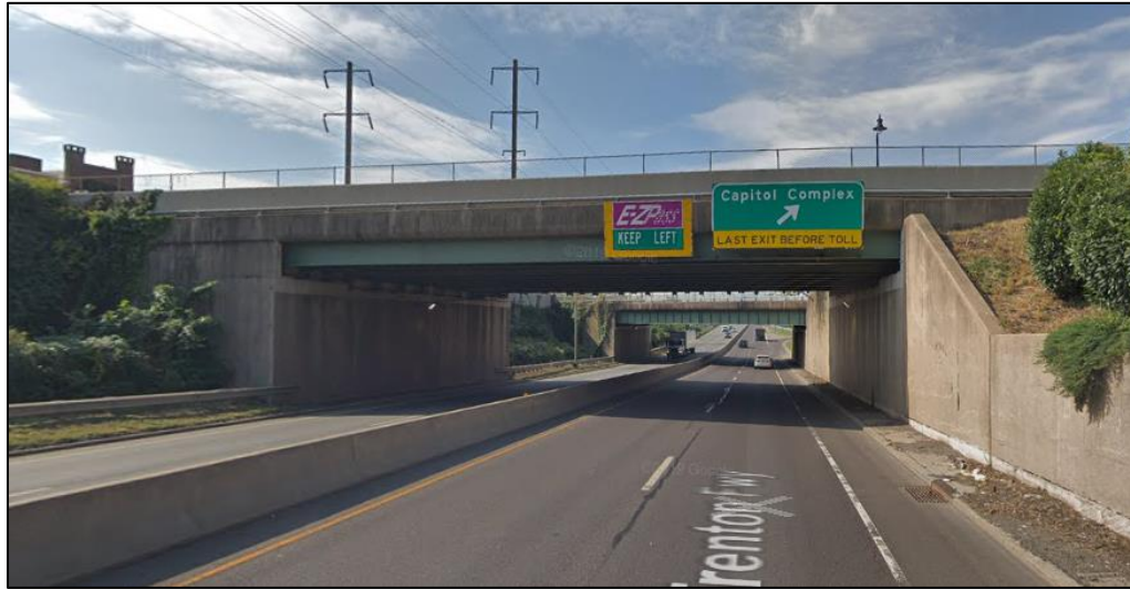
Figure 62. Southbound view of bridge from U.S. Route 1. Source: Google Street View
